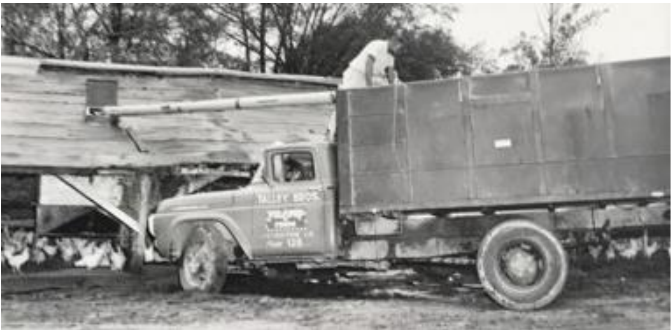
The truck could pump feed from the storage area on the bed to a hatch in the chicken house feed storage area.
